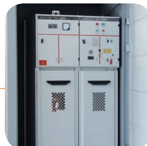
Substation high voltage chamber
